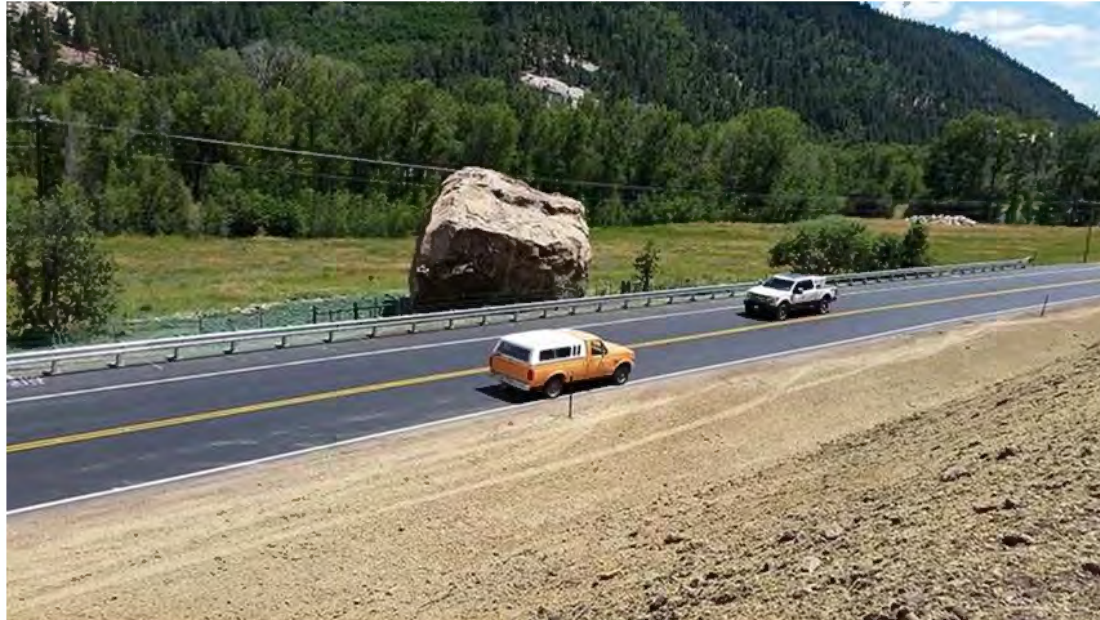
Figure 4-33 Memorial Rock and the Repaired Section of Colorado 145
